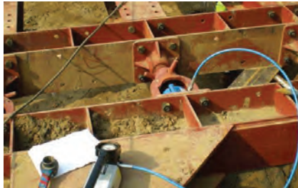
5. Jacking the corner strut
