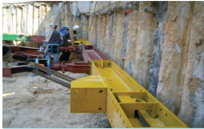
2. Placing the IPS wale
