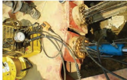
6. Jacking the PC strands
