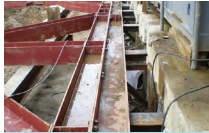
3. Welding the wale to H-pile
