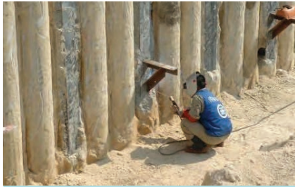
1. Excavation and placing wale support
