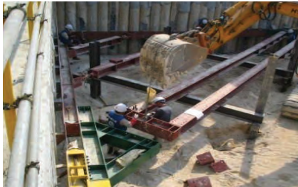
4. Placing the corner strut
